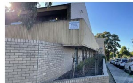
Figure 3.9 : Police station on north side Doncaster Road
