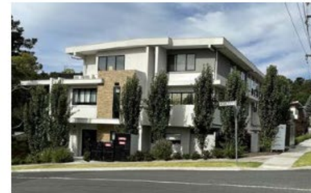
Figure 8.5 : Apartments north of Doncaster Road
