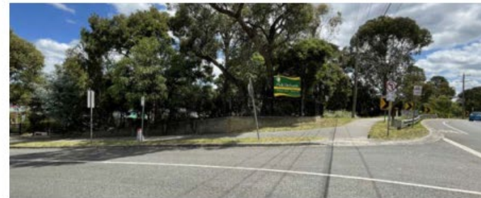
Figure 6.6 : Park Orchards Primary School
