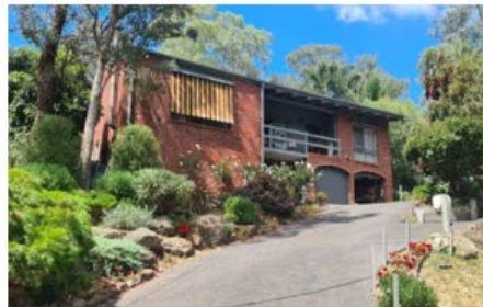
Figure 9.5 : Residence on Melbourne Hill Road
