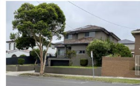
Figure 1.8 : Existing residential around Bulleen Plaza
