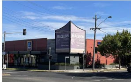
Figure 5.15 : Supermarket at the entrance of Macedon Square
