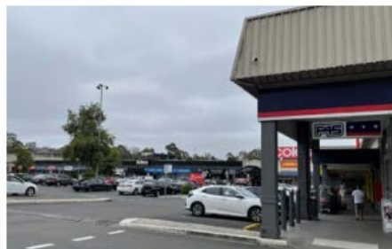
Figure 1.33 : Covered walkway along partial extent of building
