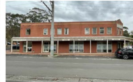
Figure 9.19 : Office building viewed from Colin Avenue
