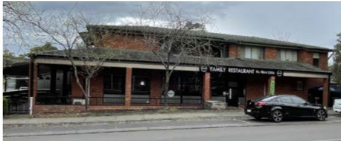
Figure 9.28 : Double storey built form from Colin Avenue
