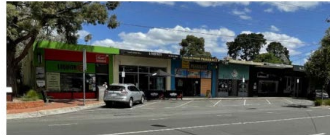
Figure 6.25: Single storey shops on Park Road
