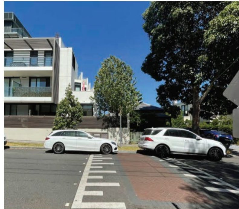
Figure 15: Built form transition at residential interface, Roseberry Street, Camberwell
