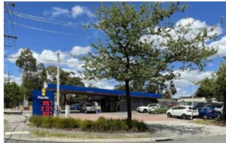
Figure 6.21: Service Station corner of Park and Hopetoun Roads
