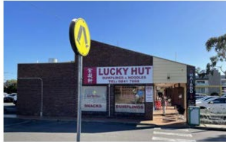
Figure 3.30 : Single storey brick building
