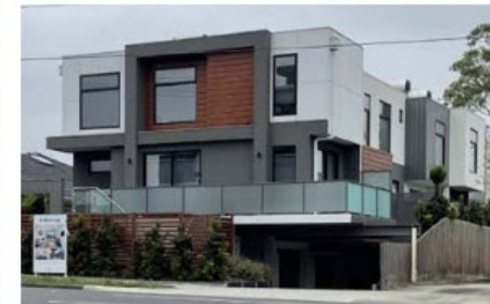
Figure 4.7 : Apartment building on Doncaster Road
