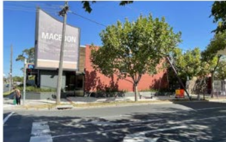
Figure 5.30 : Single storey built form of the Supermarket
