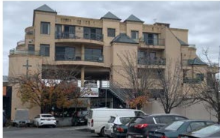
Figure 7.14 : Apartment building on the eastern end of the site
