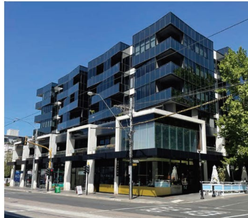
Figure 9: Mixed-use development with a defined street wall and upper levels setback, Toorak Road, South Yarra
