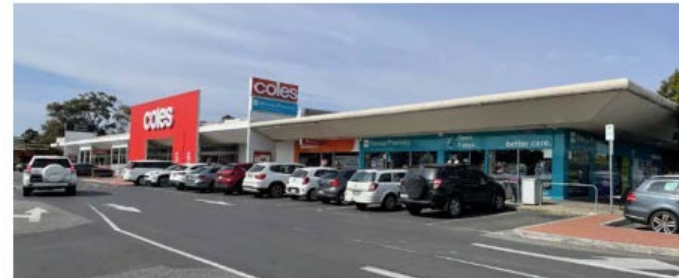
Figure 8.7 : Large supermarket to the east of Tunstall Road
