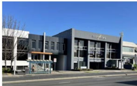
Figure 3.6 : Office buildings on the southern edge of Doncaster Road
