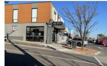
Figure 2.26 : Widened footpath with a seat
