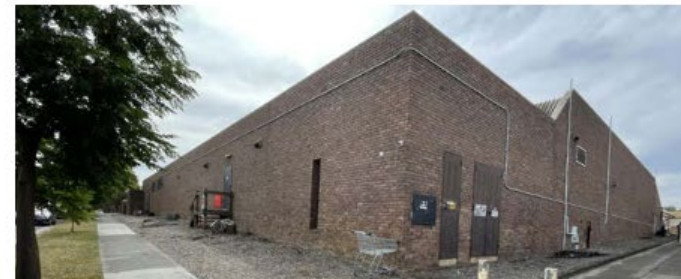
Figure 3.32 : Blank street interface south wall of Devon Plaza shopping centre
