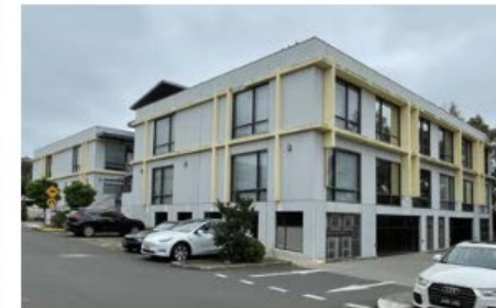
Figure 1.32 : Office building in south west corner
