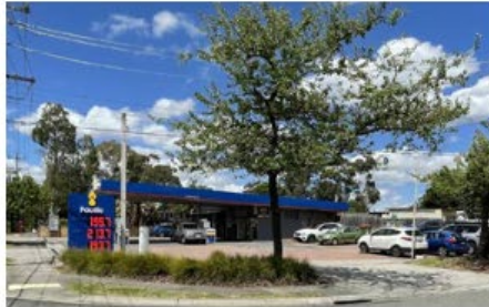
Figure 6.14 : Service Station corner of Park and Hopetoun Roads
