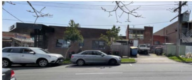
Figure 8.32: Mix of single and double storey buildings backing on to Beverley Street
