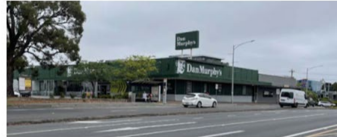
Figure 4.5 : View from Doncaster Road of Jackson Court Activity Centre
