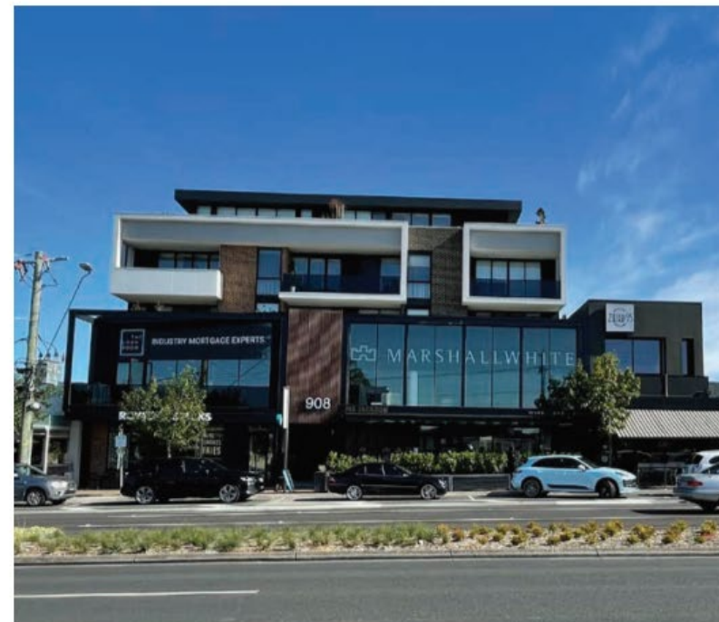
Figure 1: Doncaster Road, Doncaster East
