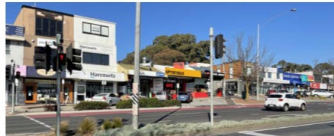
Figure 2.32 : Built form with mixed heights on the eastern edge of Blackburn Road
