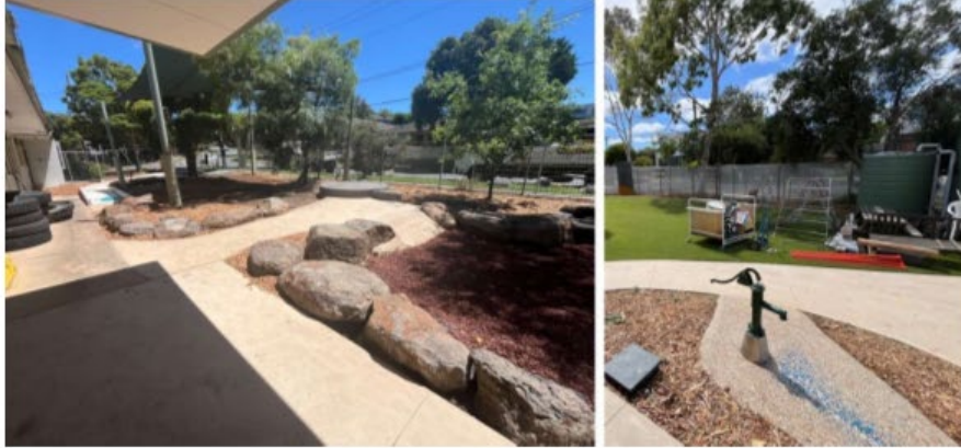
The Tunstall Square Kindergarten Expansion project is on track and nearing completion.
