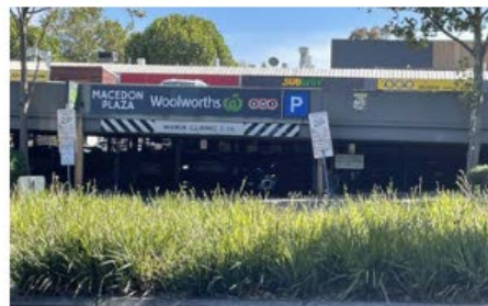
Figure 5.26 : Car park access from Manningham road to Macedon Plaza
