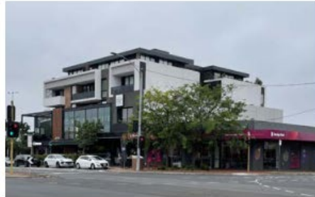
Figure 4.4 : Corner Jackson Court and Doncaster Road
