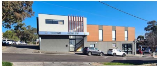
Figure 2.23 : Footpath on a steep incline Nonda Avenue
