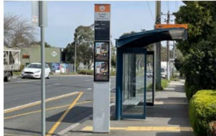
Figure 8.23 : Bus stop and footpath on Doncaster Road
