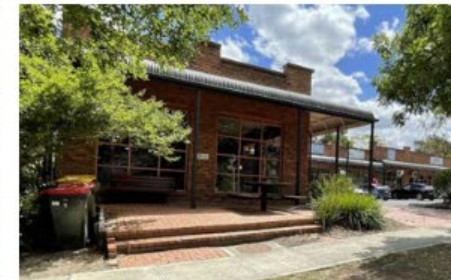
Figure 6.22: Single storey built form on Hopetoun Road with verandah
