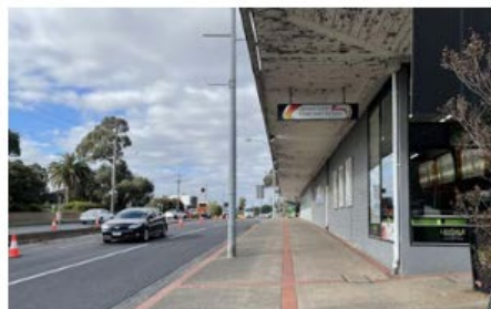
Figure 4.34 : Predominantly blank interface to Doncaster Road from Mitchell Street
