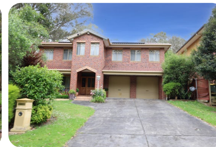
Double-storey brick dwelling with double garage - Warrandyte.
