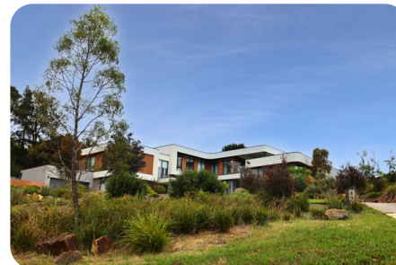
Contemporary double-storey flat roof dwelling with native garden - Donvale.
