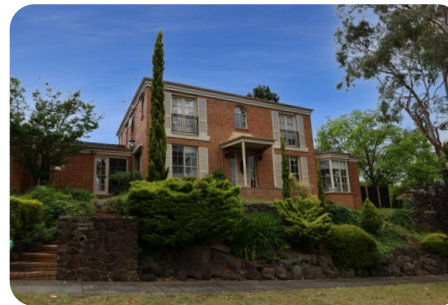
Double-storey brick dwelling - Doncaster East.
