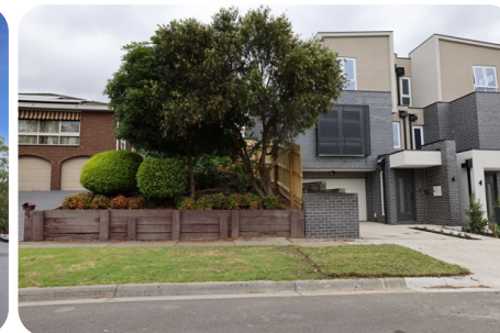
Contemporary three storey townhouse dwelling with rendered finish - Templestowe.
