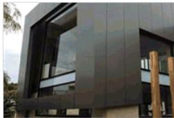
F02 SELECT METAL CLADDING WITH EXPRESSED JOINTS TO EXTERNAL WALL. COLOUR TO BE 'CHARCOAL'.
