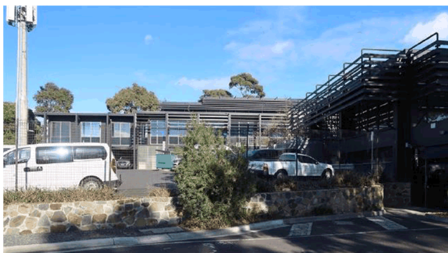
Figure 4 View of the rear (north elevation) of the Council offices showing remnants of the 1964 addition to the left and the 1977 additions to the right and the use of louvres.
